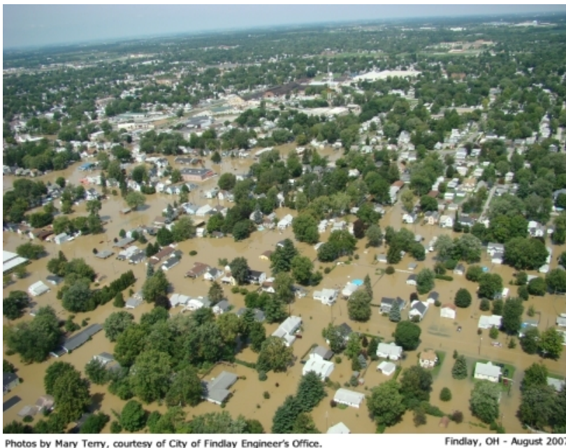
Figure 5. Extent of flooding in Findlay, Ohio, August 2007 (Source: US Geological Survey 2007)
